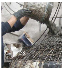
Picture 9: Filling with insulation material (Expanded Clay and cement)
