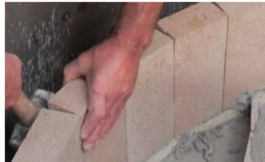
Picture 7: Hob and first circle bricks positioning
