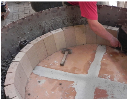
Picture 7: Hob and first circle bricks positioning
