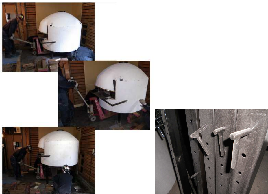
Picture 2: Example of a real installation (left) and picture of the legs with holes and “Pin stop”
